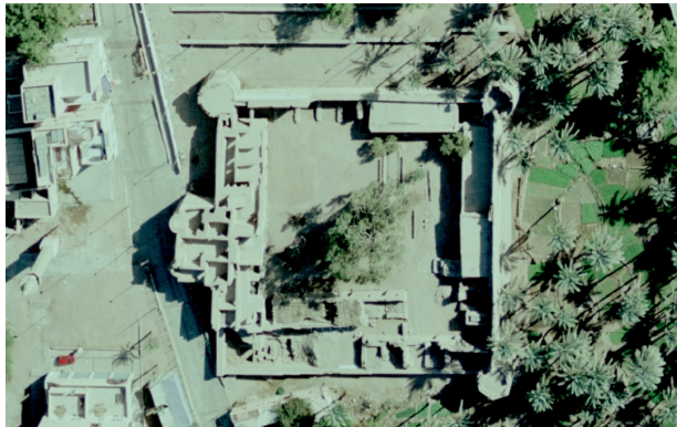
Fig. 3. Aerial view of Aqaba fort.
