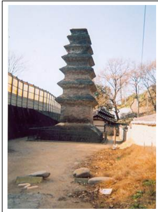
Fig. 17. Seven-story stone tower in Sinsedong, Gyeongsangbuk-do, Korea (Sin & Kim, 2006; Yoon, 2006)
